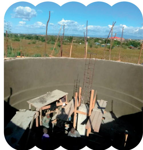
Plastering with master seal adhesive
