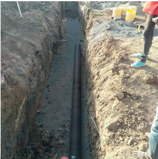
Pipe laying for road crossing
