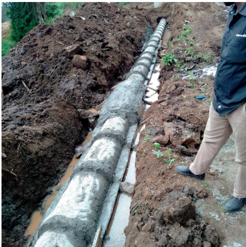
Laying of concrete pipe
