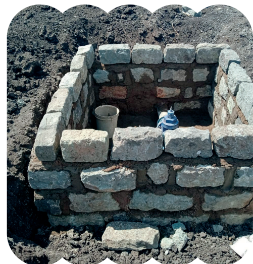
Manhole under construction
