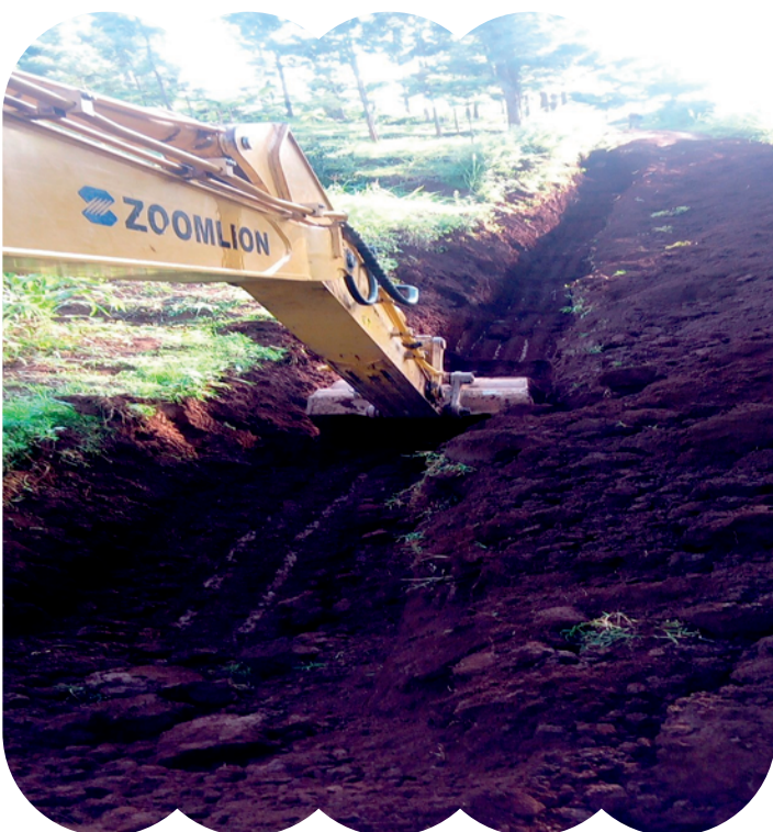
Pipeline excavation by machine
