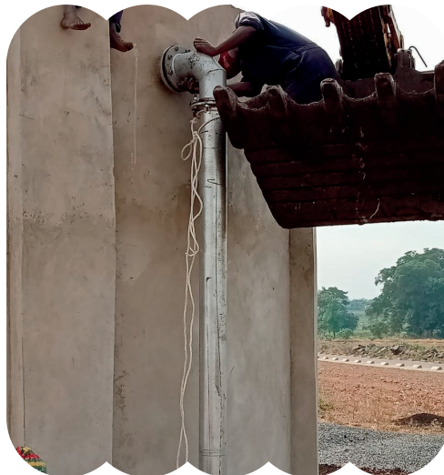
Installation of in let pipe on the farm tank
