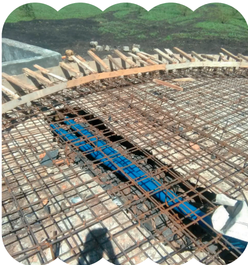
Double reinforcement of water reservoir floor
