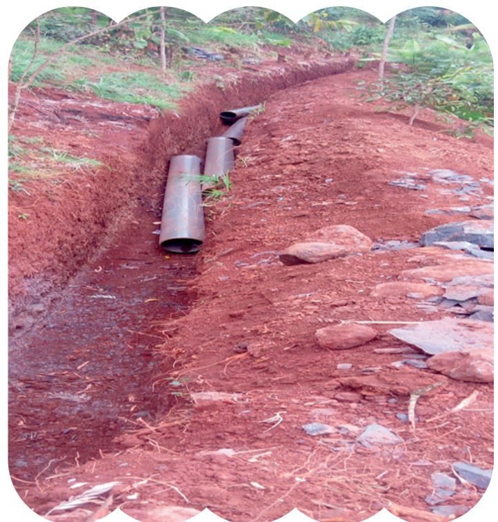
Laying off pipes in progress
