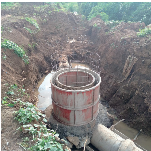
Manhole casting
