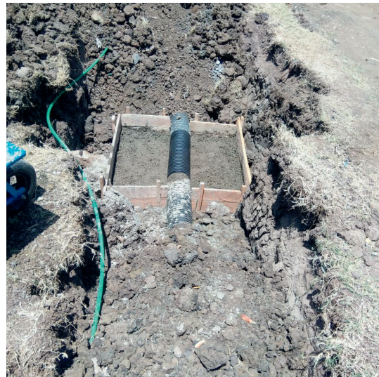
Base casting underway
