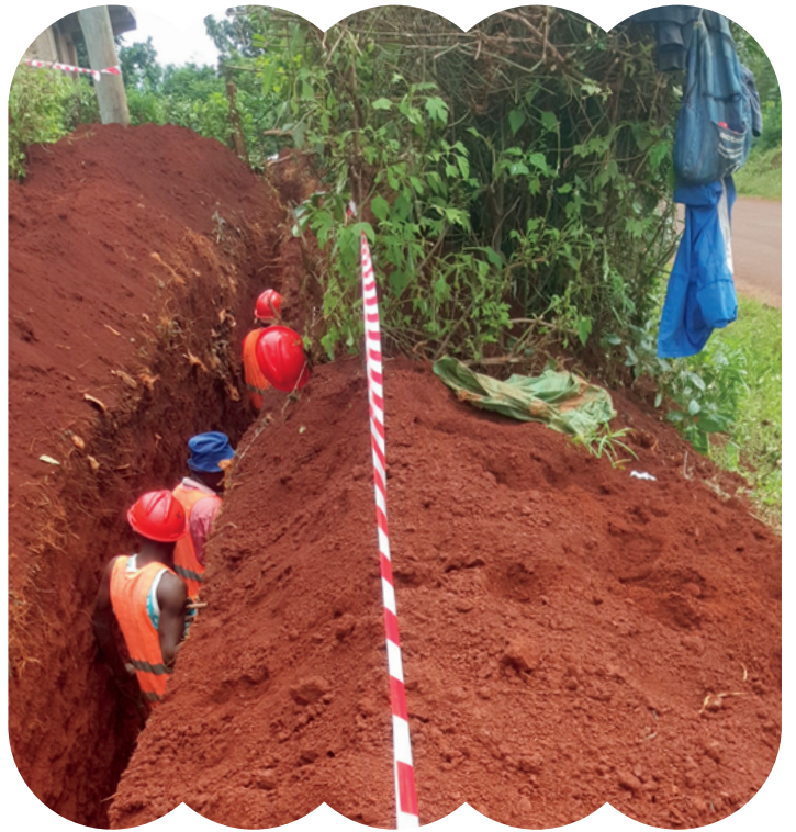
Excavation by casual labourers
