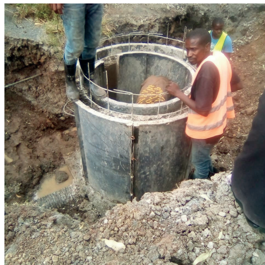
Manhole casting reinforcement
