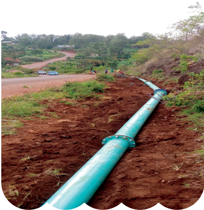
Fixing of GI pipes on a rocky pipeline area
