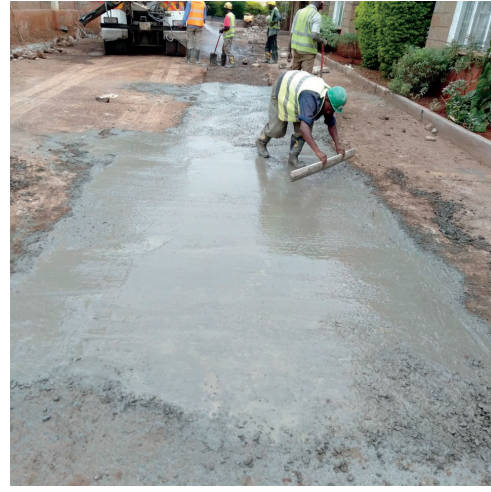
Haunching of concrete pipes
