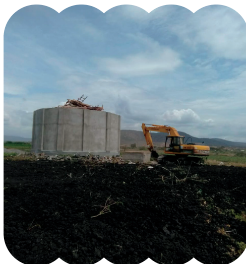
Reinstatement of the ground after construction
