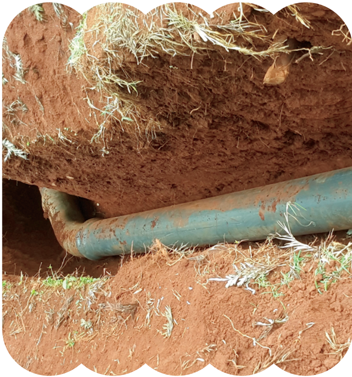
Fixing of the 11.5 degrees bend
